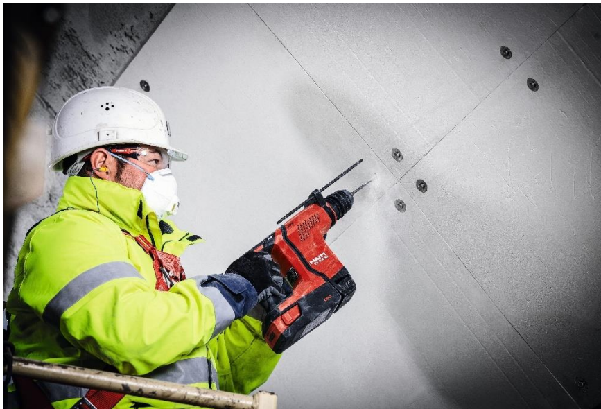
Fastening of pre-fabricated fire protection boards
